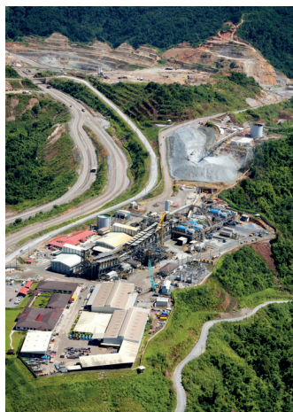
Aerial view of the Phu Kham mine
